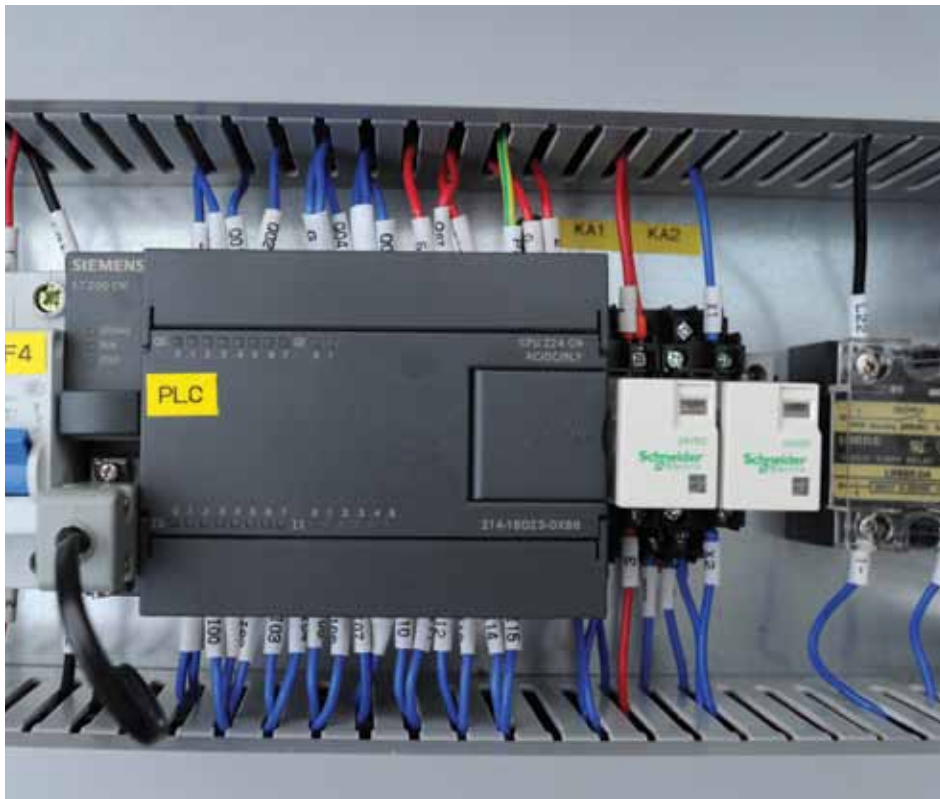
A Siemens S7-200 CN PLC control (left) and a pair of Schneider Electric's 240 VDC inductive sensors controlling the UHT (ultra-high temperature) pasteurizing line.
